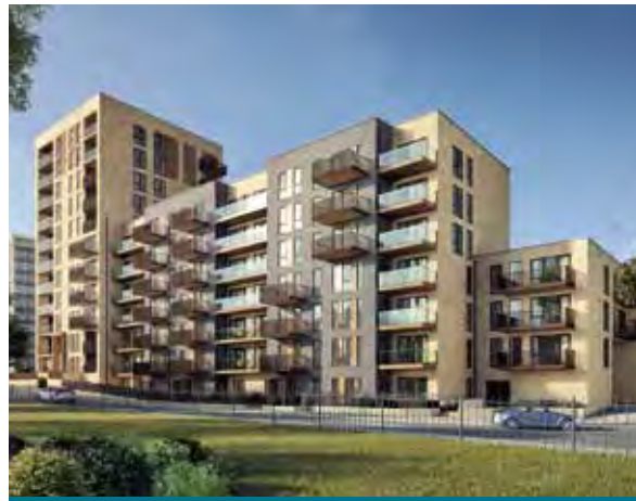
View of Phoenix from the south west.
